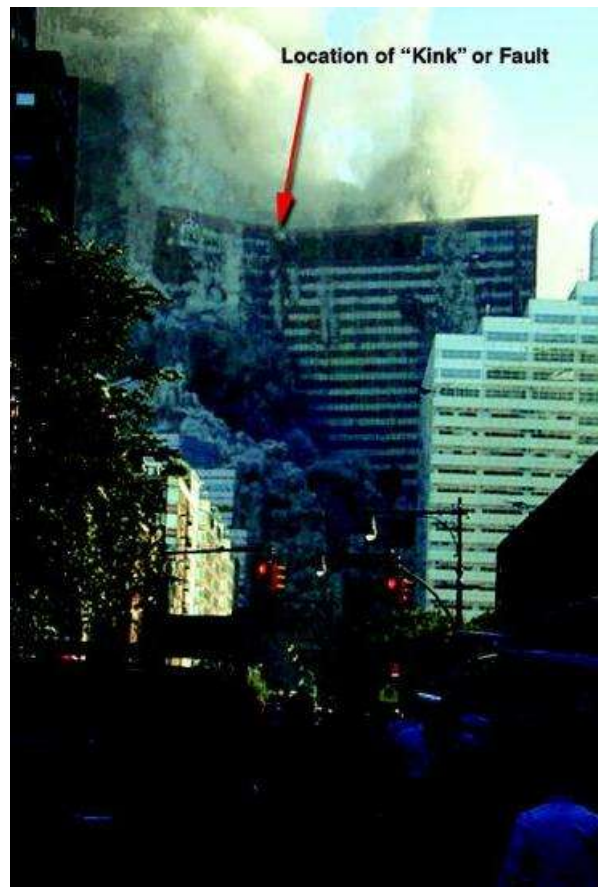
WTC7 collapsing – the structure is descending to the ground maintaining its shape, completely symmetrically, which give us a proof of a deliberate demolition
